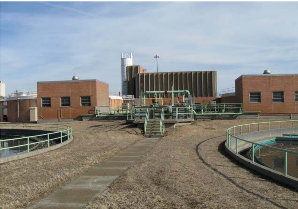
Figure 2 – Grit Basin (Center) and Grit Handling Superstructure (Looking North)
