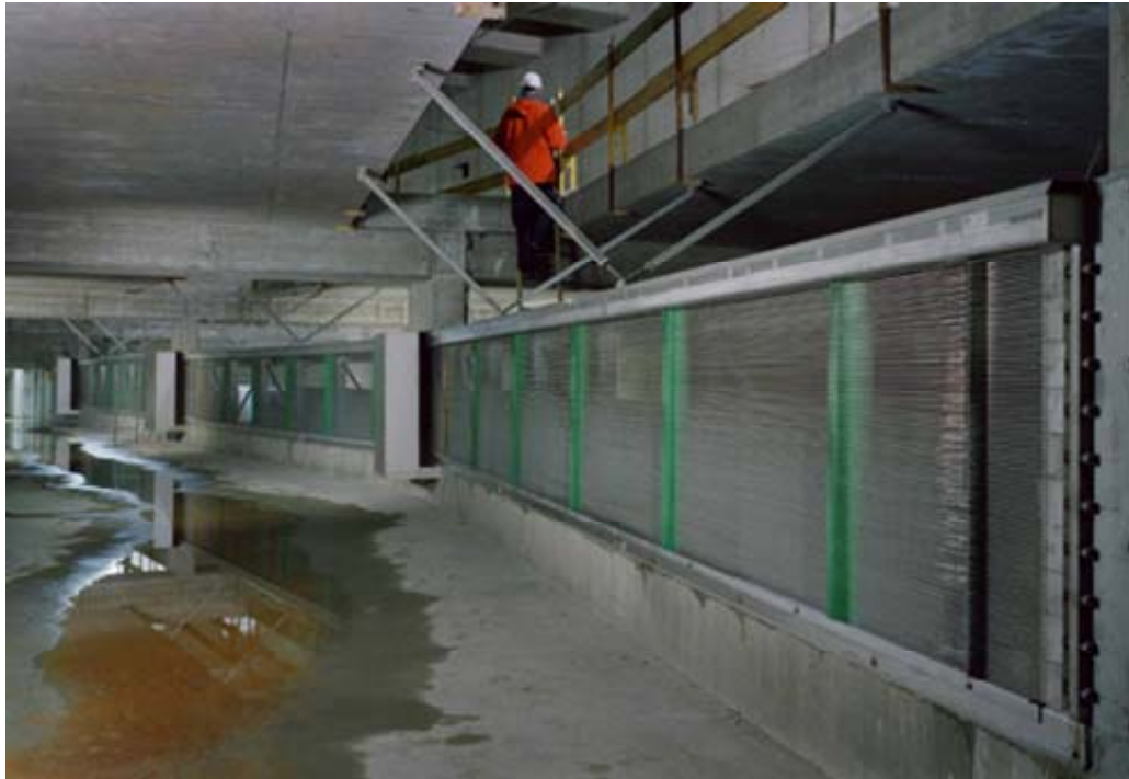
Figure 11 – Specialty CSO Bar Screen – Vertical Configuration
